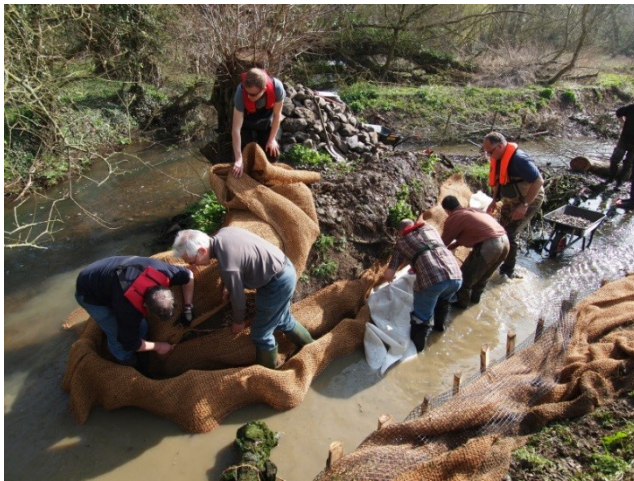
The first Loddon Rivers Week - volunteers and partners building a fish and wildlife bypass channel
